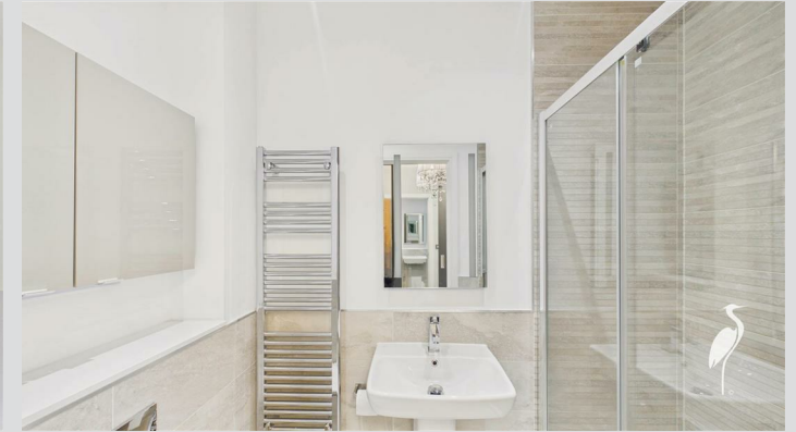
Low level WC with concealed cistern, washbasin and walk in shower cubicle.
